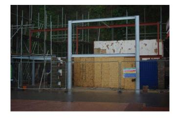
With the steels in and the scaffolding finished the front is also now protected from the elements with sheeting and we've been able to have Building Control back to ok the latest work which they did yesterday (22<sup>nd</sup>). We are now starting to put the wooden framework in for the first floor and we are expecting the roof trusses by mid-January.
