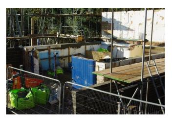
We now have some of the new ground floor walls and a new concrete ring beam in place, this was followed by the steel framework which finished going in on Monday (19<sup>th</sup>).
